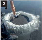
Remove gel residues from the work area and clean the surface.
