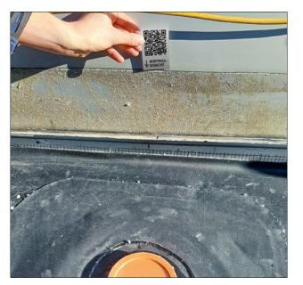
The position plaque should be visibly attached to the façade or terrace covering.
